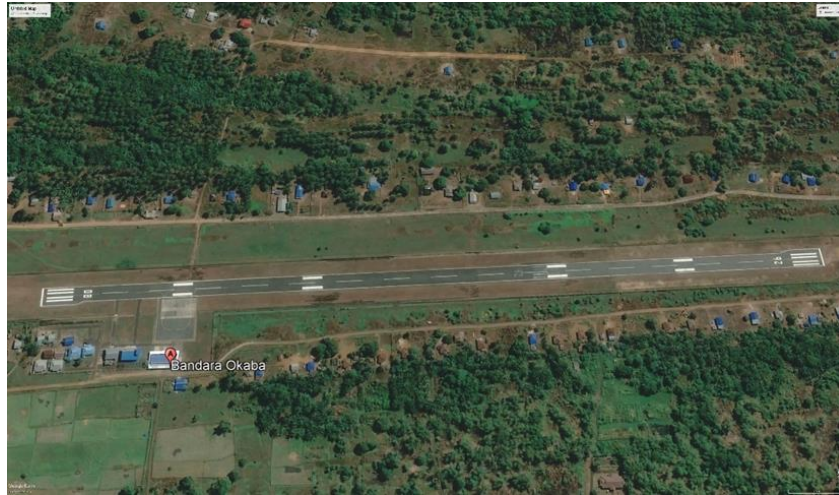
Figure 2. Image of research location
